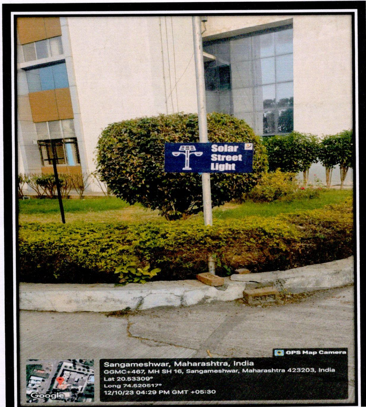
Solar Street Light
